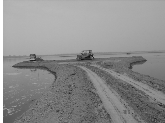
Coffer Dam construction
